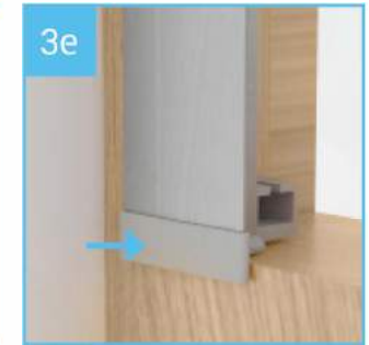
3e Position the bottom of siderail tight against edge of window.
